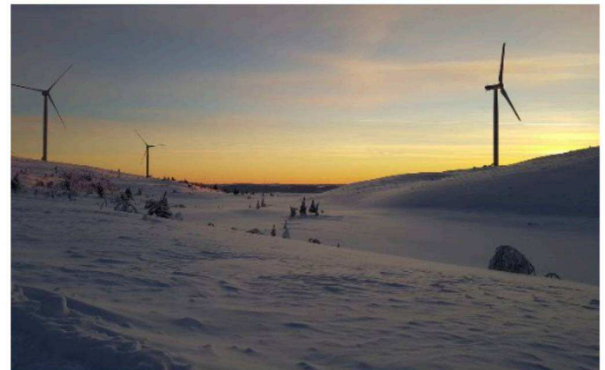
The blades of wind turbines are often damaged by ice that releases from the plant when the blades spin.
