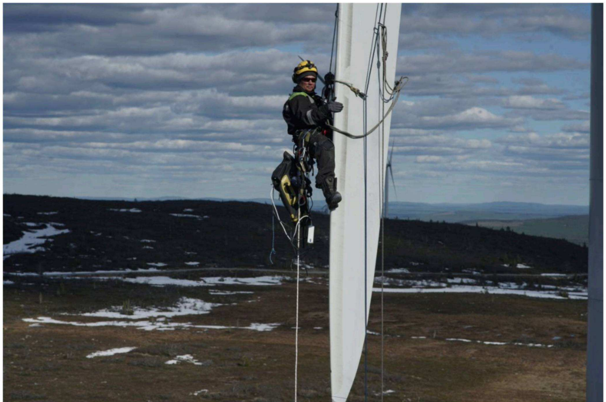
Greger Nilsson has recently tested an epoxy glue that hardens in minus degrees to repair damaged wing blades.
